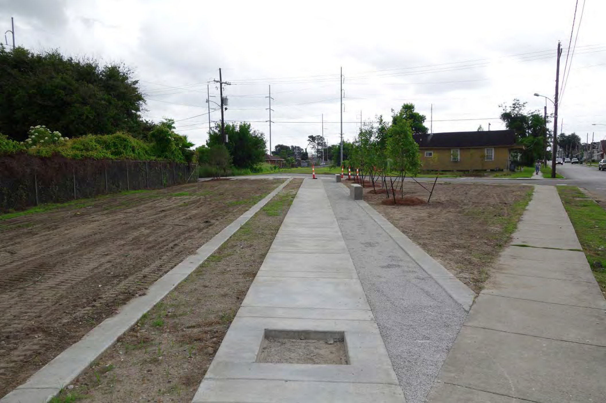
View of Phase 1 Construction Looking East from Forshey Street
