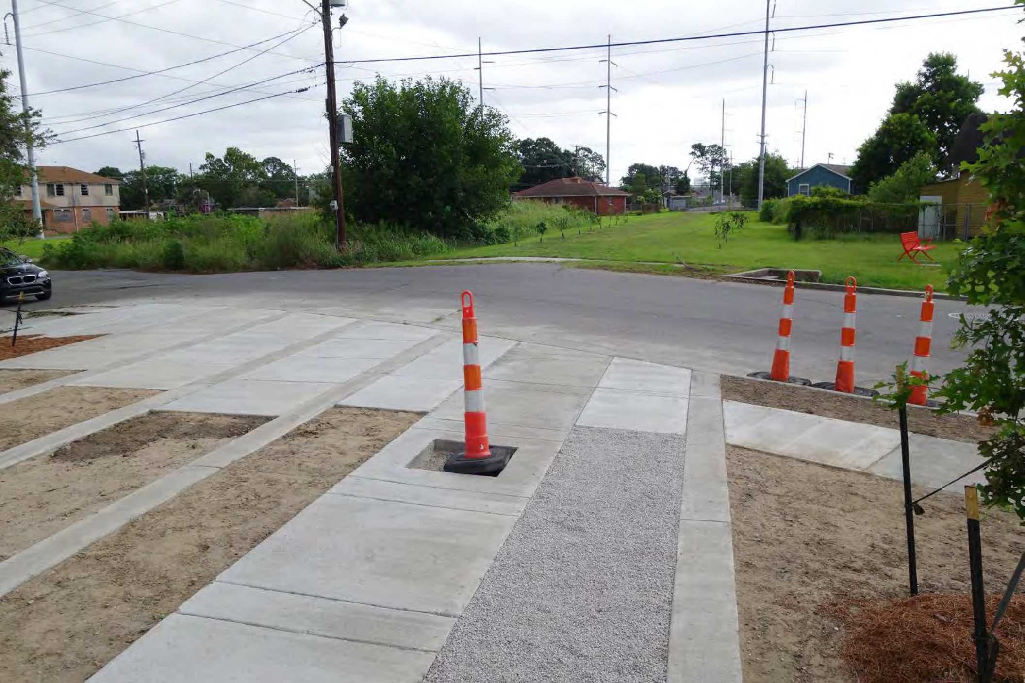
View of Phase 1 Construction Looking East- NORA Water Retention Garden is at Right
