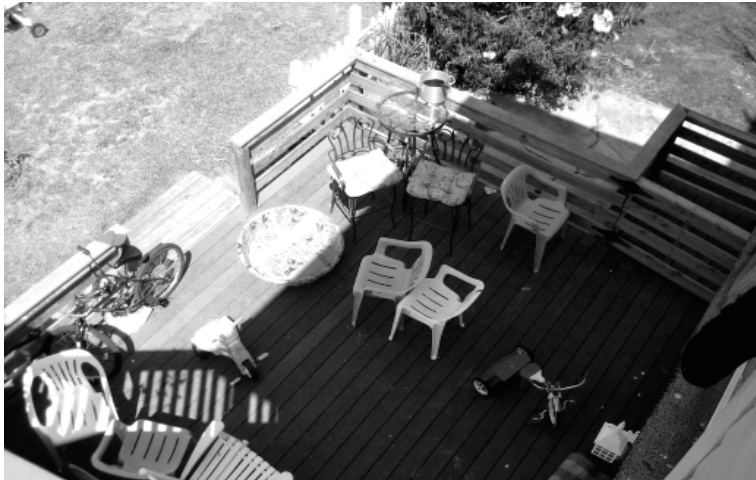
DISMANTLING THE DECK : OCTOBER 1 - OCTOBER 4
