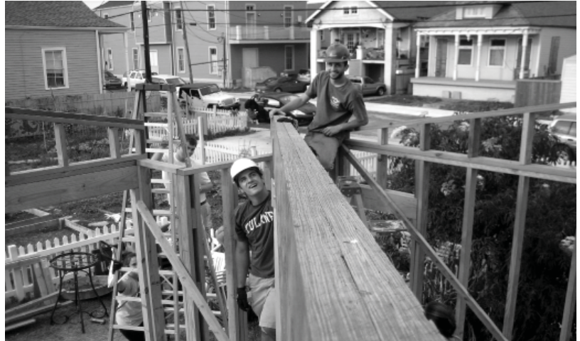
COPLANAR ROOF FRAMING: OCTOBER 28 - NOVEMBER 11
