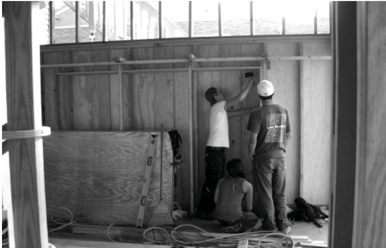
FINISHING THE INTERIOR : NOVEMBER 17 - DECEMBER 15
