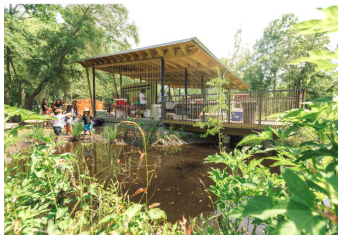
Figure 3: Top to Bottom: Students working on the construction of the outdoor teaching space; Final project in use at Sugar Roots Farm; The final project as a functioning ecosystem and education space with children catching crawfish in the water retention pond.
