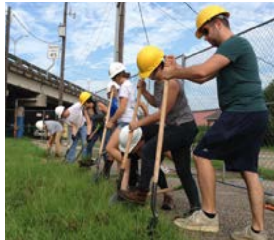
PARISITE SKATE PARK Initial rendering (above), designers meeting to talk about a model (far right), and students starting construction (near right)
