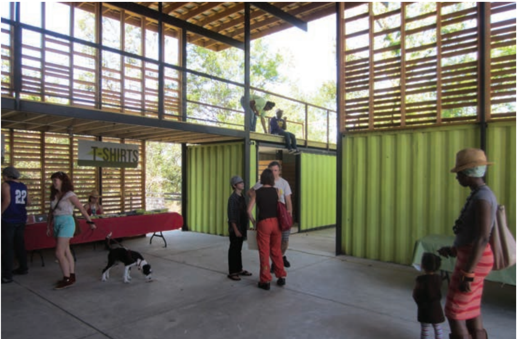
Grow Dat's teaching campus is a series of shipping containers housing teaching and farm support spaces, and providing the structural support for large covered outdoor spaces
