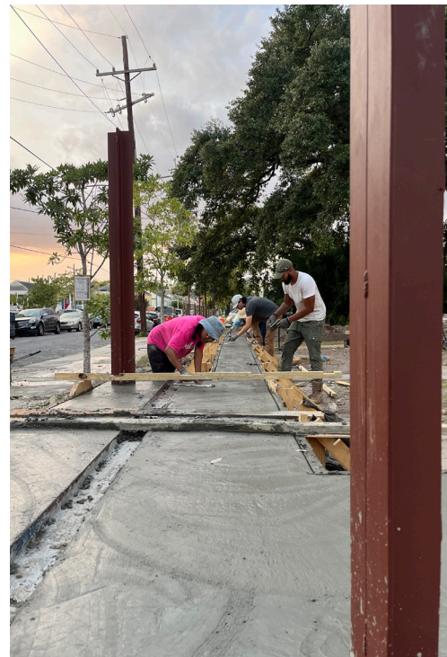
PLINTH The plinth was designed to support public seating in the outdoor classroom, and also includes an imbedded trough which channels runoff water directly to a waiting rain garden.
