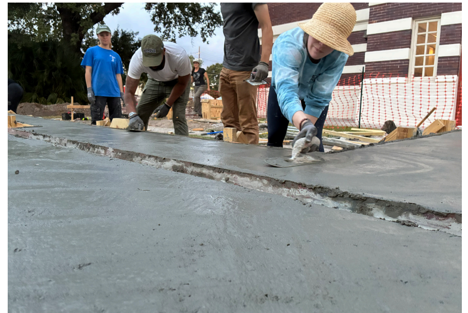
PLINTH The plinth was designed to support public seating in the outdoor classroom, and also includes an imbedded trough which channels runoff water directly to a waiting rain garden.
