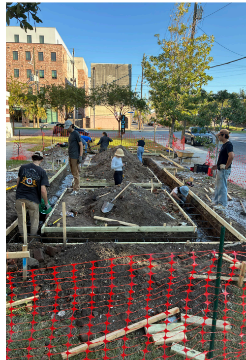
FOUNDATION The foundation was designed to anchor columns and meet code-required wind-lift regulations for the pavilion roof. Students recovered a large number of bricks during excavation and were able to reuse some of them elsewhere in the project.
