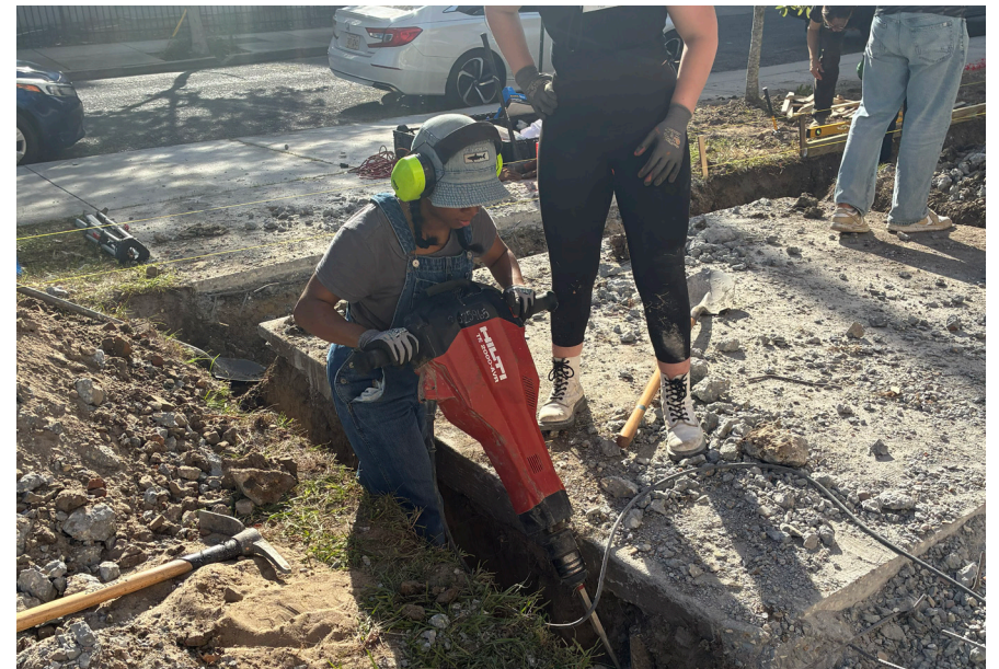
FOUNDATION The foundation was designed to anchor columns and meet code-required wind-lift regulations for the pavilion roof. Students recovered a large number of bricks during excavation and were able to reuse some of them elsewhere in the project.
