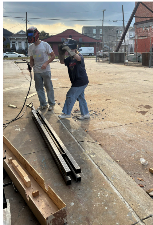
COLUMNS Unique "quad" columns were designed and fabricated at Small Center, then installed on site. Their open structure contributes to the light and airy quality of the overall design.
