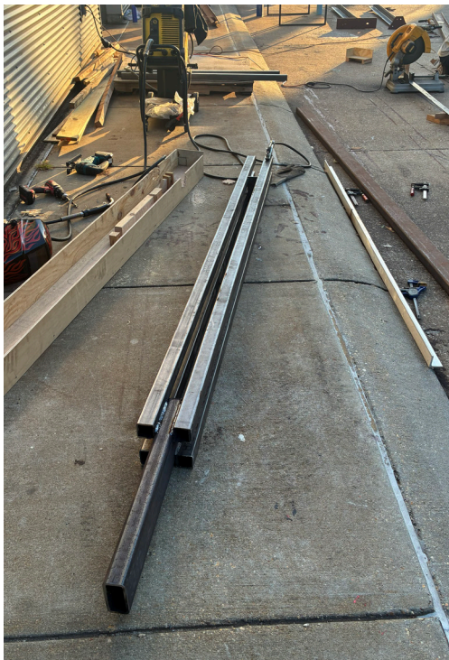
COLUMNS Unique "quad" columns were designed and fabricated at Small Center, then installed on site. Their open structure contributes to the light and airy quality of the overall design.
