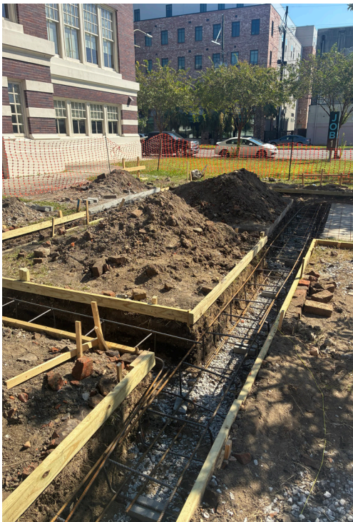
FOUNDATION The foundation was designed to anchor columns and meet code-required wind-lift regulations for the pavilion roof. Students recovered a large number of bricks during excavation and were able to reuse some of them elsewhere in the project.
