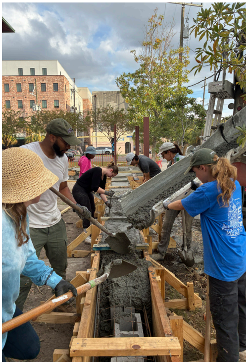
PLINTH The plinth was designed to support public seating in the outdoor classroom, and also includes an imbedded trough which channels runoff water directly to a waiting rain garden.
