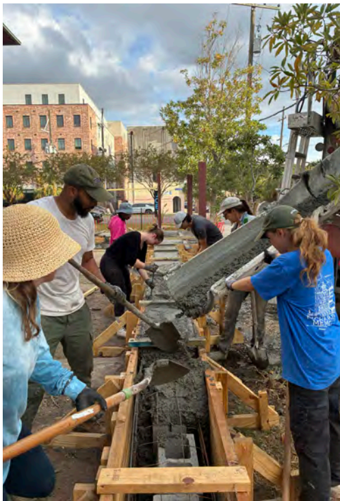
PLINTH The plinth was designed to support public seating in the outdoor classroom, and also includes an imbedded trough which channels runoff water directly to a waiting rain garden. Cedar formwork used for the pour were retained and repurposed as raised planter beds.
