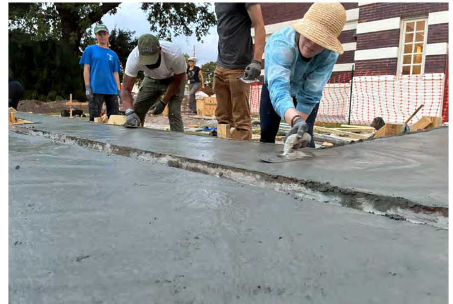
PLINTH The plinth was designed to support public seating in the outdoor classroom, and also includes an imbedded trough which channels runoff water directly to a waiting rain garden. Cedar formwork used for the pour were retained and repurposed as raised planter beds.
