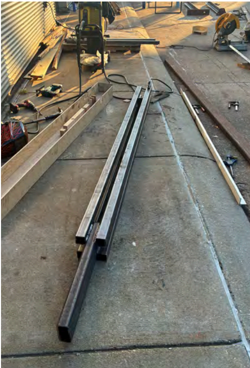
COLUMNS Unique “quad” columns were designed and fabricated at Small Center, then installed on site. Their open structure contributes to the light and airy quality of the overall design, and were designed to receive the beams and trusses in an interlocking structure.
