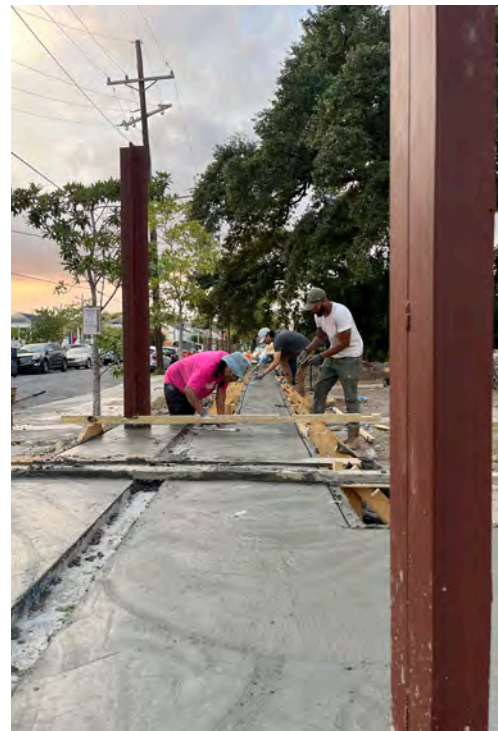
PLINTH The plinth was designed to support public seating in the outdoor classroom, and also includes an imbedded trough which channels runoff water directly to a waiting rain garden. Cedar formwork used for the pour were retained and repurposed as raised planter beds.
